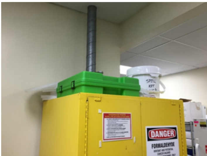
Figure 34 Ventilated Flammable Gas Cabinets
